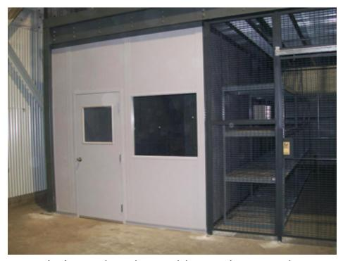
ground floor and second level storage lockers using wire partitions and a mezzanine system. As seen in the photos, WireCrafters enclosed the mezzanine to create a secure area.
