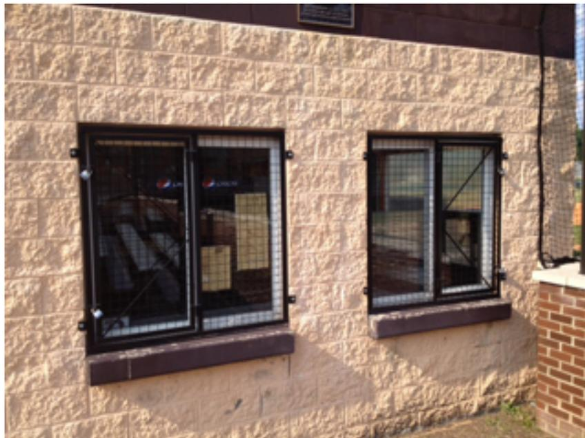
The welded wire window guards were outfitted with two padlock lugs which were welded on the top and bottom of the window guards for added security. WireCrafters then provided an outdoor grade, black powder coat finish to the window guarding in order to withstand the unpredictable weather (such as rain, heat, and snow) of the Ohio Valley.
