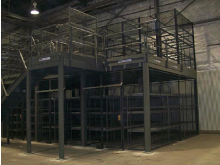
front of the adjacent wall panel. In many cases hinged doors would be used but they must have room to swing into an aisle way, and for the NAS there wasn't enough room. The doors were placed in the center of the security enclosure so shelving units could be accessed on either side of the wire partition
