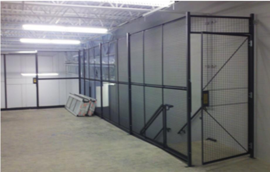
Typically, secure wire partitions are built with a 3 inch sweep space at the bottom. However, since the secure wire partitions in this application were installed on a second level, a kick plate was put in place to keep small parts from rolling under the partition
