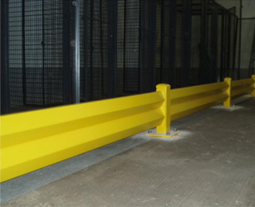
WireCrafters GuardRail was installed in one foot increments from 1'-0" wide to 10'-0" wide sections to achieve the different lengths required inside the distribution facility. The bright safety yellow rails were bolted to 4" square uprights using hardware that was provided; including the 3/4" x 4-1/4" floor anchors.
